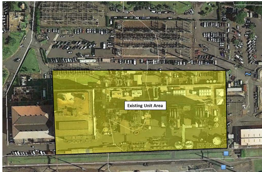
Figure 5-14. Existing Waiau Generating Unit Area
