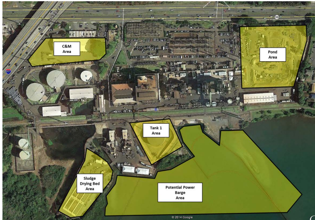
Figure 5-15. Other Areas at the Waiau Generating Station
