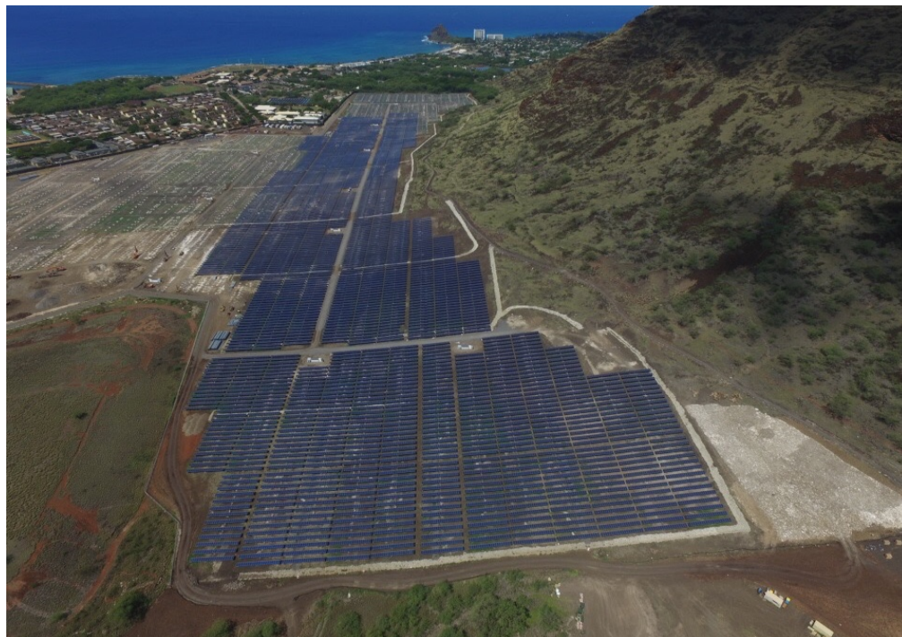
Figure H-3. Waianae Grid-Scale Solar Facility on O'ahu (broad under-construction viewpoint)
