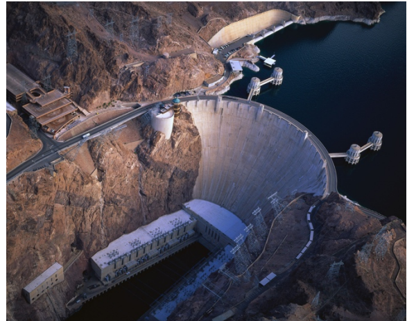
Figure 22. Hoover Dam Power Plant
