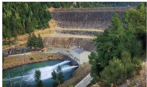
Figure 21. Tieton Hydropower Project
