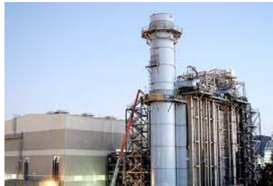
Figure 14. Magnolia Power Plant
