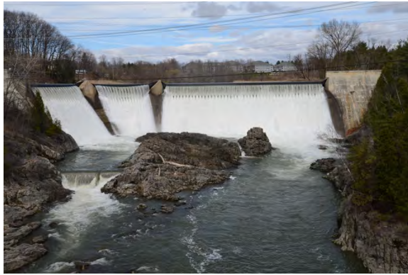
Figure 5-4. Essex #19 Hydro Station
