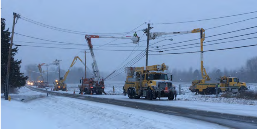
Figure 6-6. Line Crew Restoring a Storm-Related Outage
