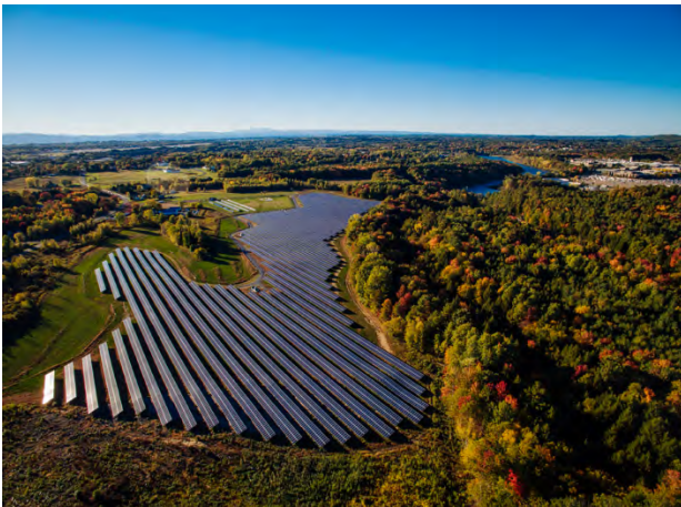
Figure 5-15. Williston Solar Facility
