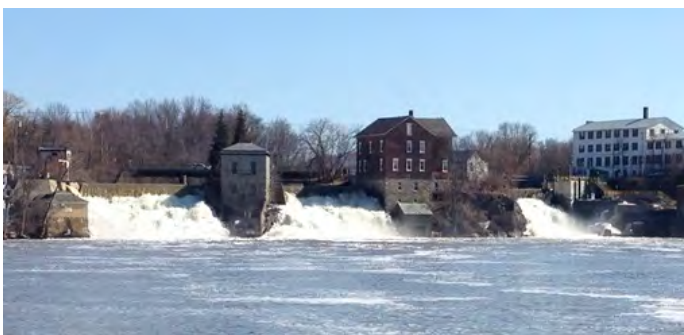
Figure 5-8. Vergennes Hydro Facility
