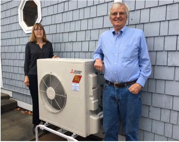
Figure 2-4. A Customer with Their Ductless Heat Pump
