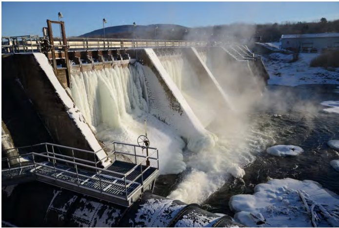
Figure 5-3. Clarks Falls Hydro, Milton
