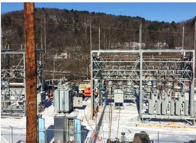
Figure C-4. White River Junction Substation During Construction
