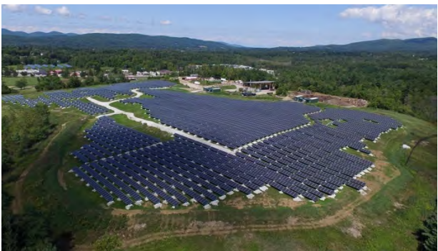
Figure 5-10. Stafford Hill Solar Facility
