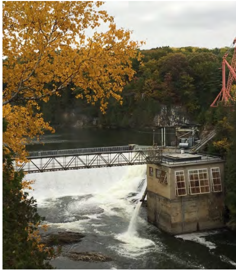
Figure 5-6. Gorge #18 Hydro Facility
