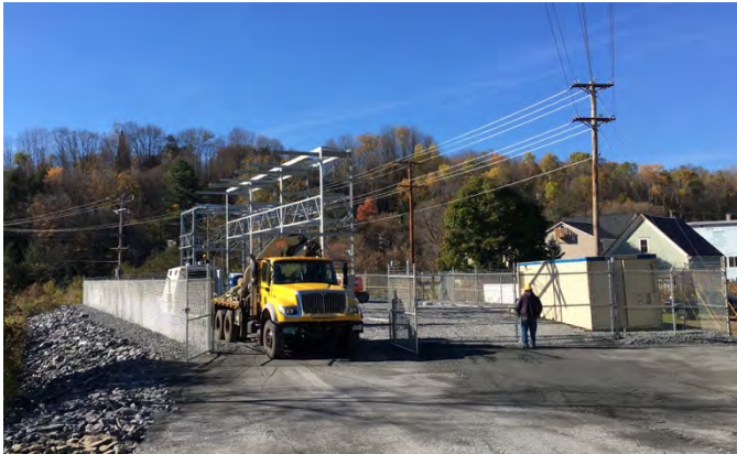
Figure C-5. Ongoing Construction of New Barre South End Substation
