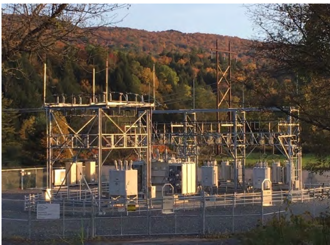
Figure C-3. Waterbury Substation: Relocated and Replaced
